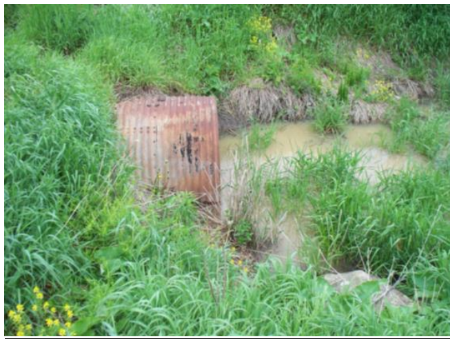
Figure 6.9 Culvert in poor condition on Rayment Drain in Subwatershed 5
