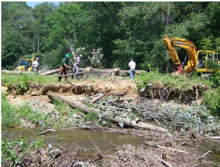
Figure 6.5 Large woody material removal and bank stabilization in Columbus County Park
