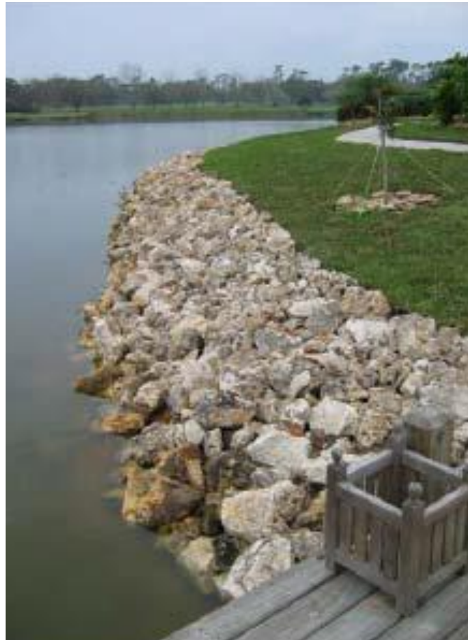
Figure 6.7 Example of riprap shoreline stabilization practices
