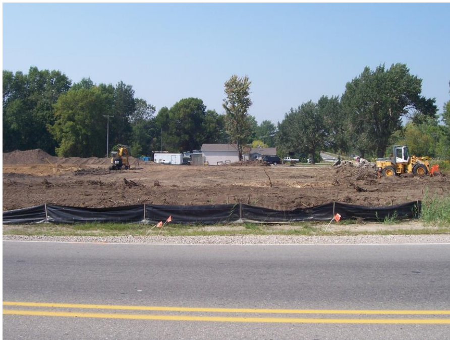
Figure 6.23 A silt fence is an example of a Soil Erosion and Sedimentation Control BMP (Source: SCCHD)
