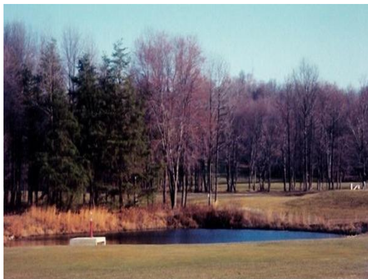
Figure 6.10 Example of a wet detention pond to detain stormwater (Source: US EPA)
