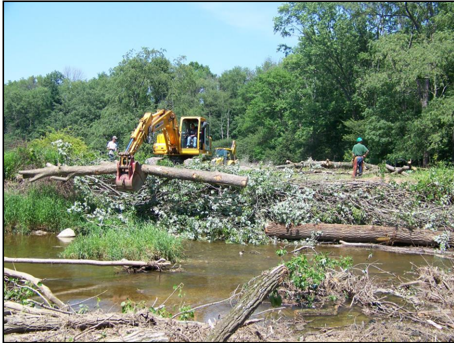
Figure 5.4 SCC PARC streambank stabilization demonstration project using large woody material from the Belle River, Columbus County Park
