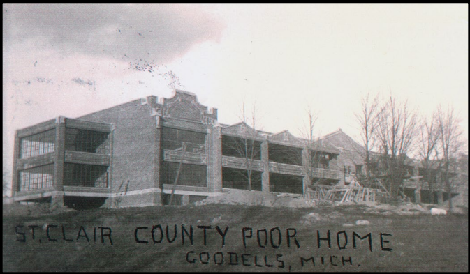
The new infirmary under construction in 1914. Looking northeast.
