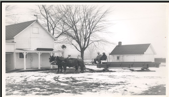
Some of the outbuildings. The building to the left served as a general store for residents.
